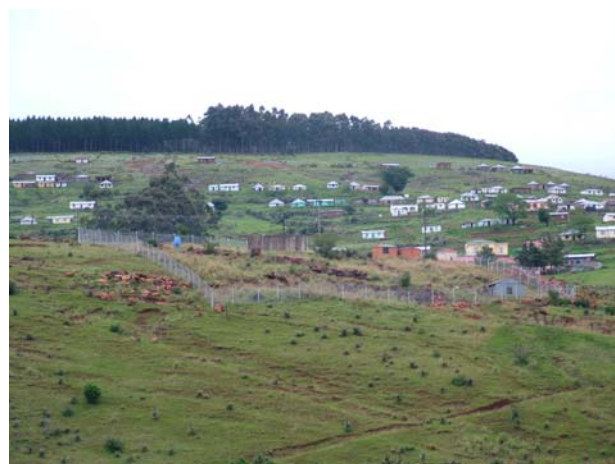
Figure 1 Upper Mnyameni (Treatment Plant in Foreground Enclosure)
